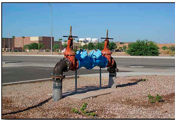
Figure 22-47 Commercial OS&Y Water Valve
