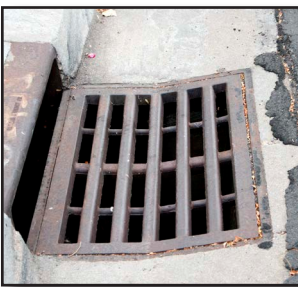
Figure 22-53 Storm Drain Grate
