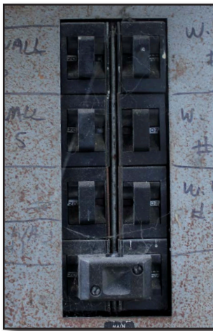
Figure 22-25 Push Button Type Circuit Breaker
