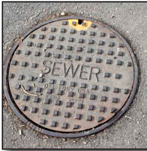
Figure 22-51 Sewer System Manhole Cover
