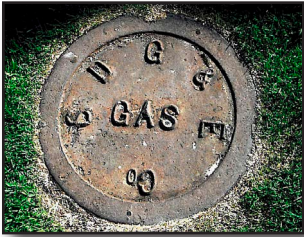
Figure 22-34 Curb Gas Valve
