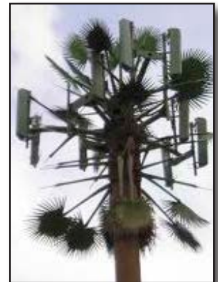
Figure 22-59 Cell Phone Towers
