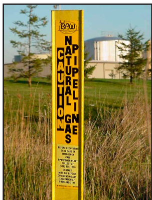
Figure 22-32 Gas Transmission Line Marker
