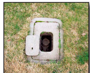
Figure 22-46 Meter Valve
