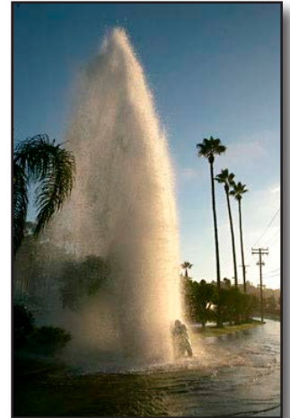
Figure 22-49 Knocked Off Fire Hydrant
