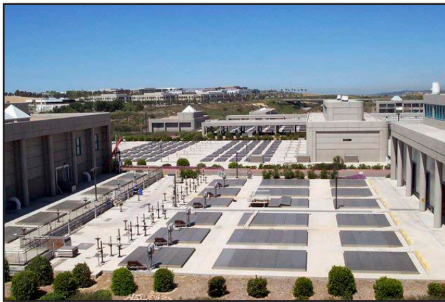
Figure 22-52 North City Water Reclamation Plant
