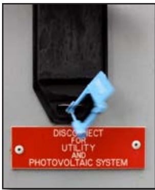
Figure 22-28 Photovoltaic Disconnect
